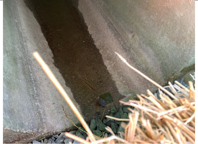
29 Gundalow -1 (Drainage Area)
