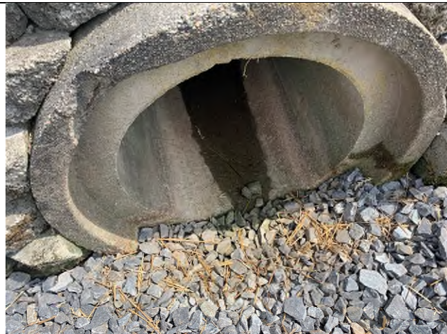
29 Gundalow - 1 (Drainage Area)
