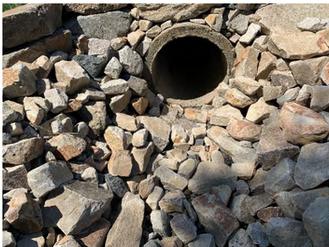
64 Gundalow - 1 (Drainage Course)
