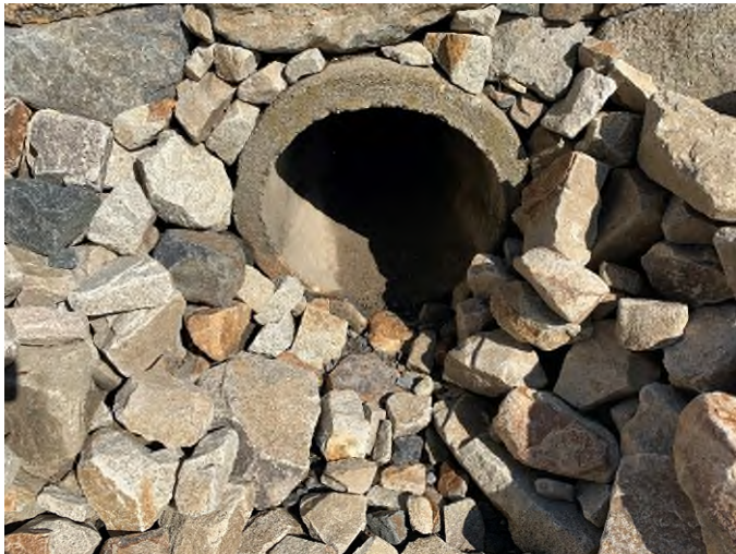
64 Gundalow - 1 (Drainage Course)
