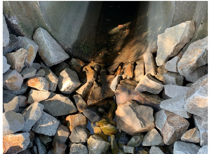
64 Gundalow - 2 (Drainage Course)
