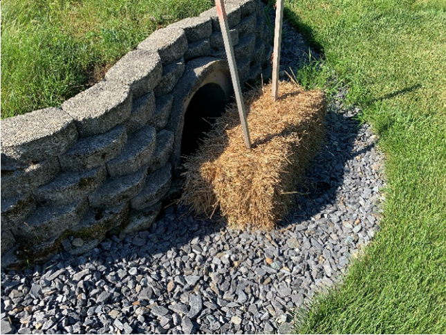
29 Gundalow -1 (Drainage Area)
