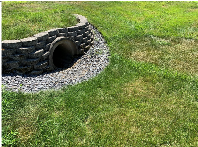
29 Gundalow - 1 (Drainage Area)
