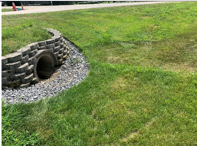
29 Gundalow - 1 (Drainage Area)
