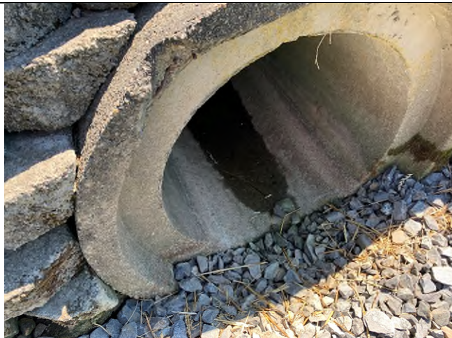
29 Gundalow - 1 (Drainage Area)
